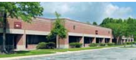
Hauptsitz USA headquarter USA, Brecksville, Ohio
